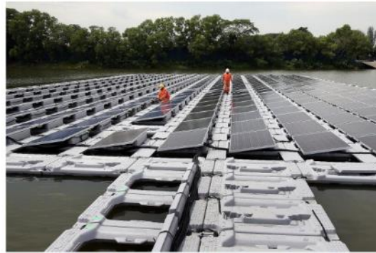
A floating solar photovoltaic cell test-bed in Tengeh Reservoir in Tuas in 2016. While such panels cost more to install, they are up to 16 per cent more efficient because the water's cooling effect helps reduce thermal losses and extend their life, according to the Solar Energy Research Institute of Singapore. ST FILE PHOTO.
