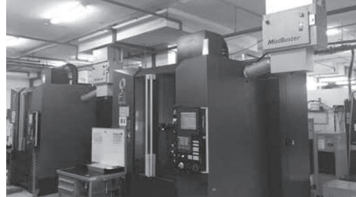
Mist Buster Air Filtration Systems on machines
