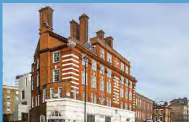
Expanded into the UK residential market with the acquisition of the former Westminster Fire Station for redevelopment into a mixed-use development in the City of Westminster, central London
