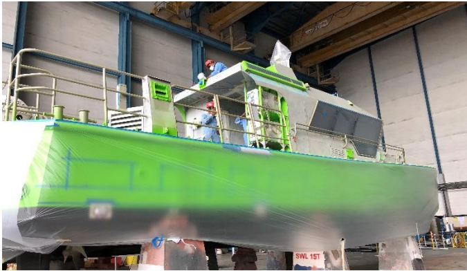
"Penguin Tenaga" under construction
