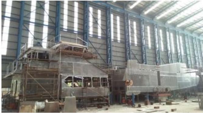
WindFlex-27 under construction
