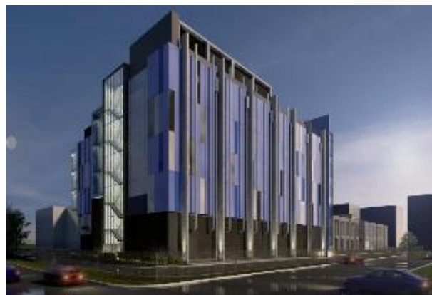
Intellicentre 3 East Data Centre
