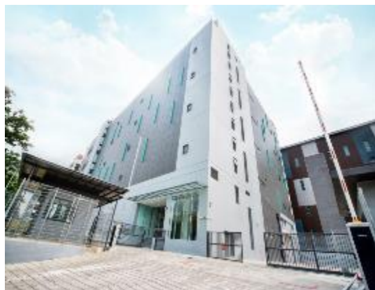
Keppel DC Singapore 5
