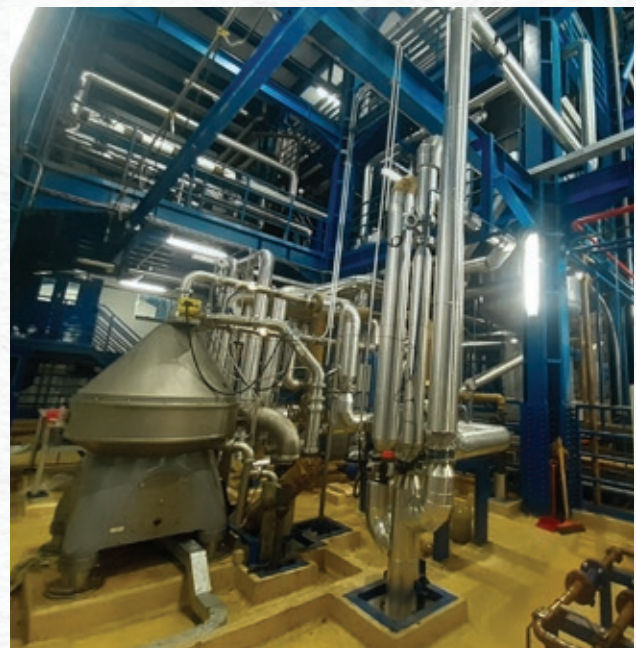
New production line at Tanjung Priok refinery
