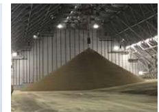
Indoor coal storage area
