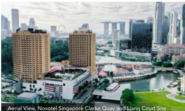
Aerial View, Novotel Singapore Clarke Quay and Liang Court Site
