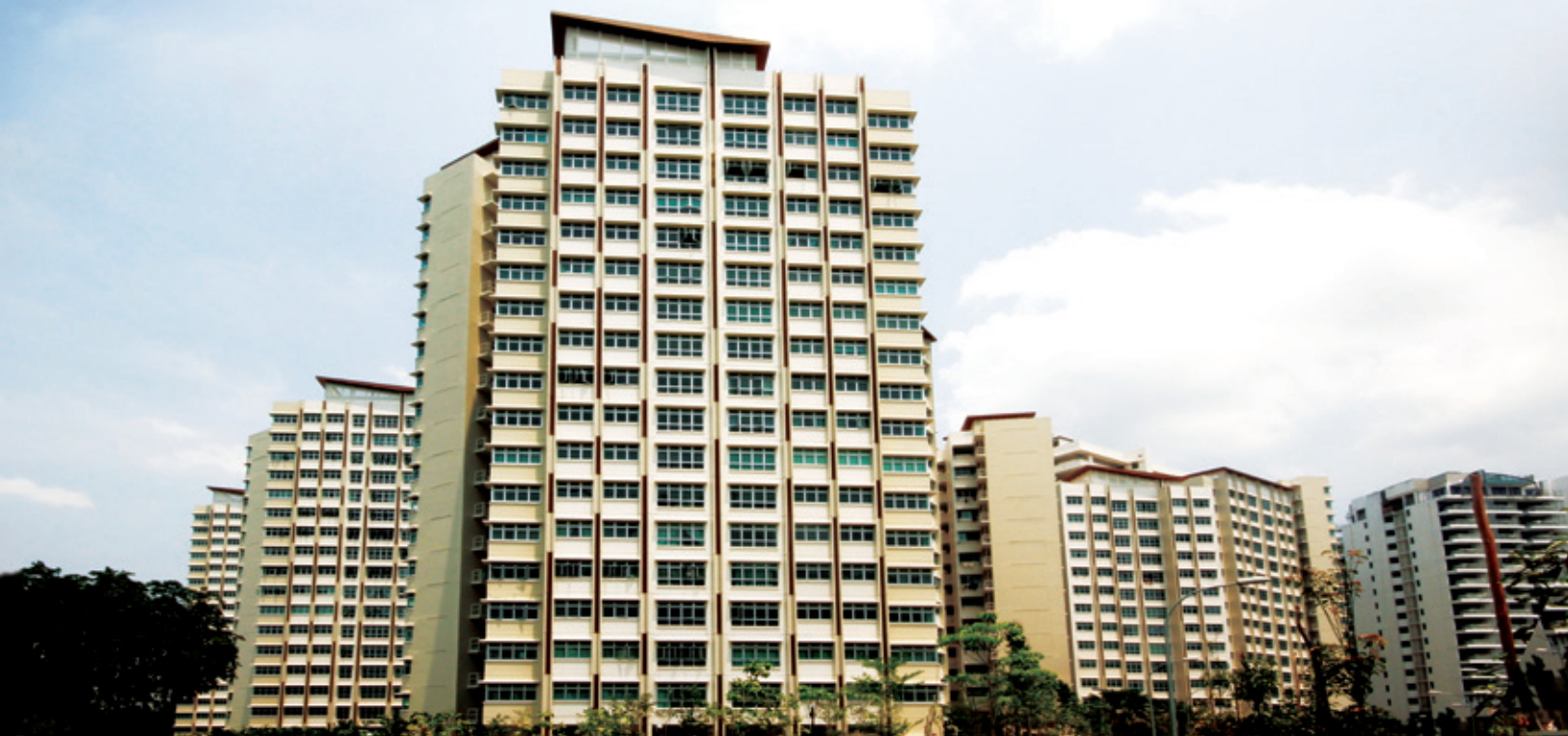
Hougang N4C17, Singapore - a HDB project completed in 2014
