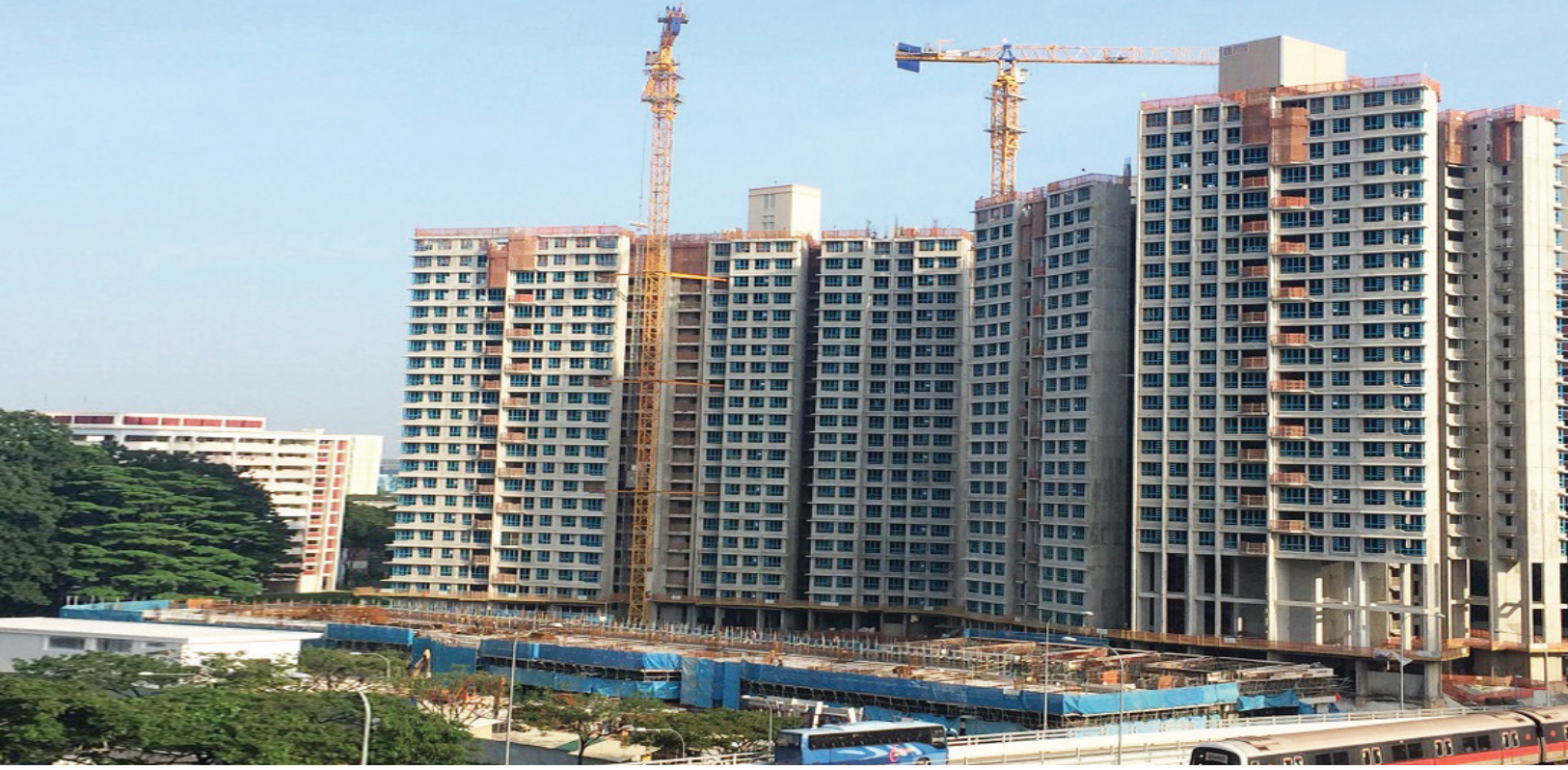
Bukit Batok N1C13 & N2C23, Singapore - a HDB project under construction
