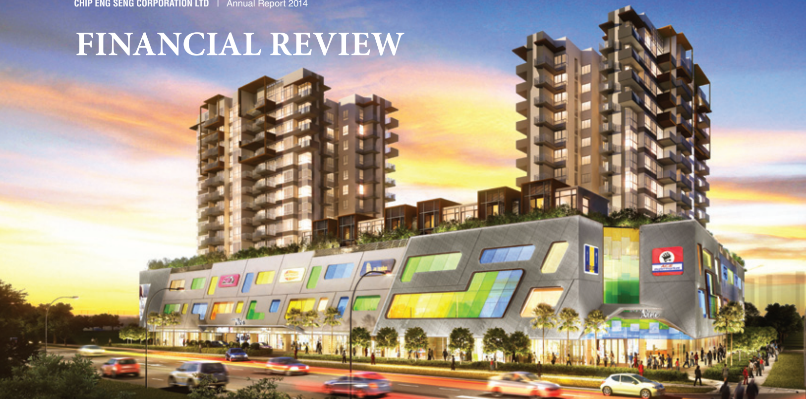
Junction Nine & Nine Residences, Singapore - a mixed residential and retail development under construction
