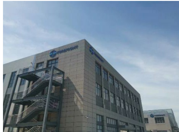
Plant Extension in Changzhou, China
