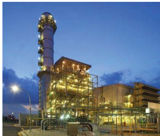
Keppel Merlimau Cogen plant
