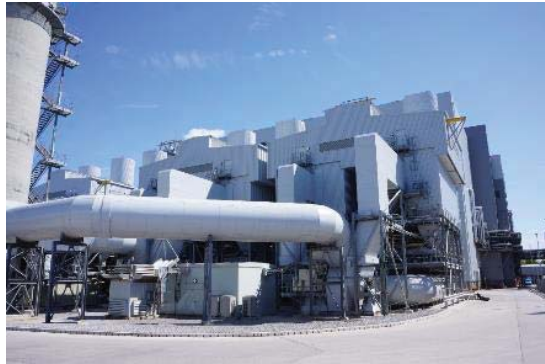
Greater Manchester Energy-from-Waste Plant, the UK
