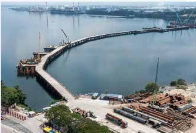
JB-SG RTS Link Marine Viaduct project
