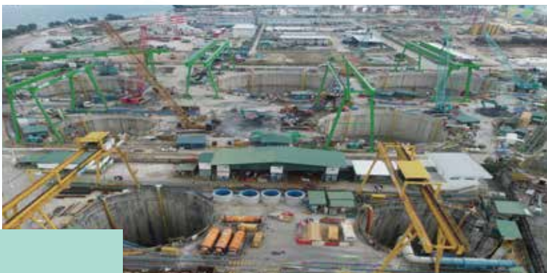
TWRP-C2A project (top 5 shafts) and DTSS-T08 project (bottom 2 shafts)
