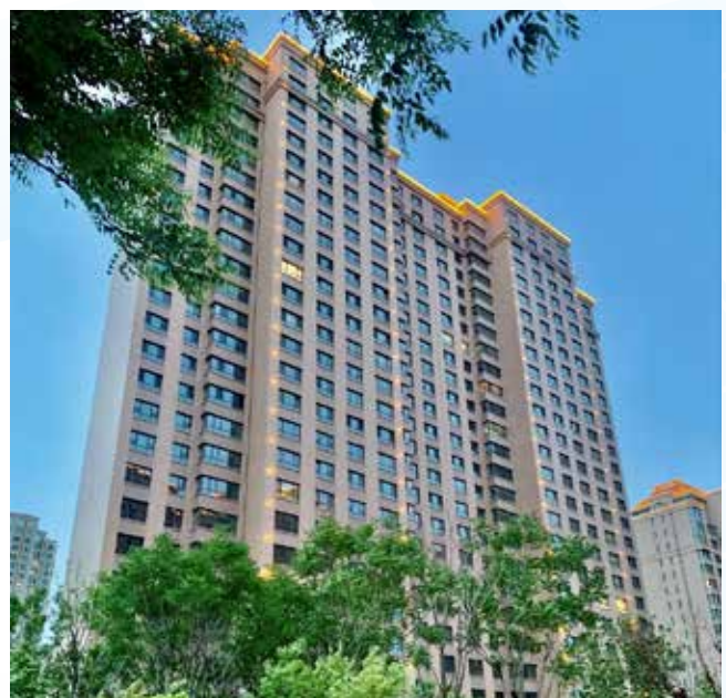
Tangshan Nanhu Eco-City project
