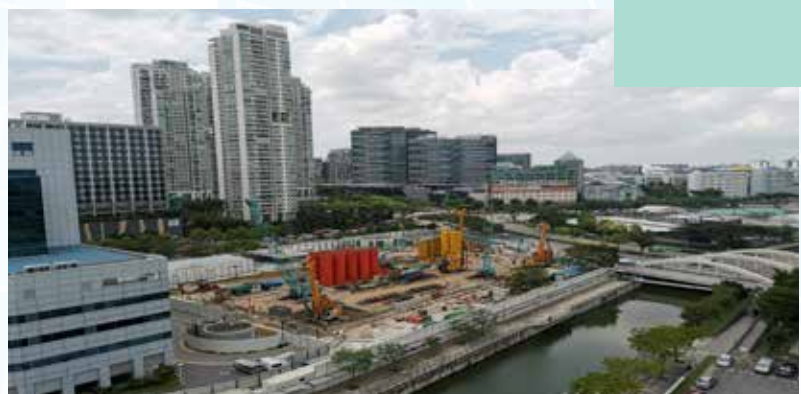
Expansion and retrofitting of ICA
