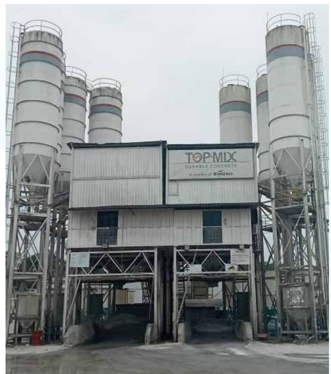
TMM batching plant
