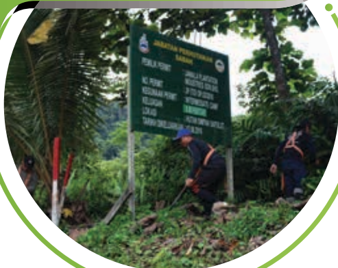
SURVEY DEPARTMENT Survey Crew demarcating the boundary for O.P site
