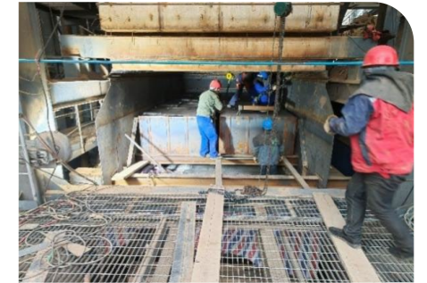
>>> Installation of SCR system
