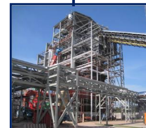
MAJU INTAN BIOMASS POWER
