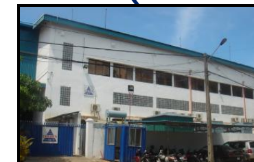
SIHANOUKVILLE THERMAL POWER
