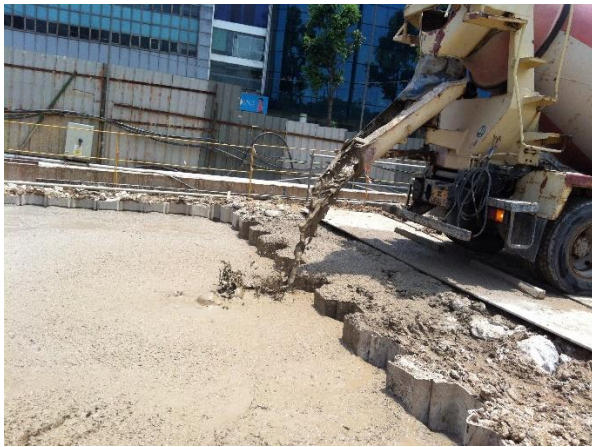
Eco-friendly LSS used to stabilise the earth
