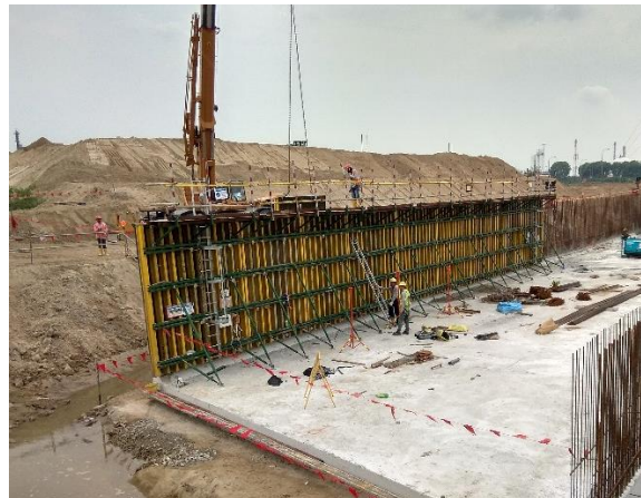
System formwork used for drain construction
