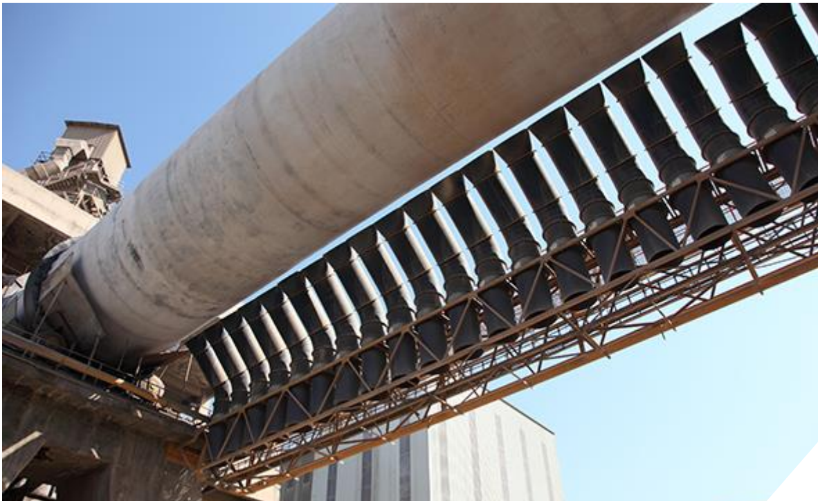
Mill Close up – Matola Plant – Mozambique
