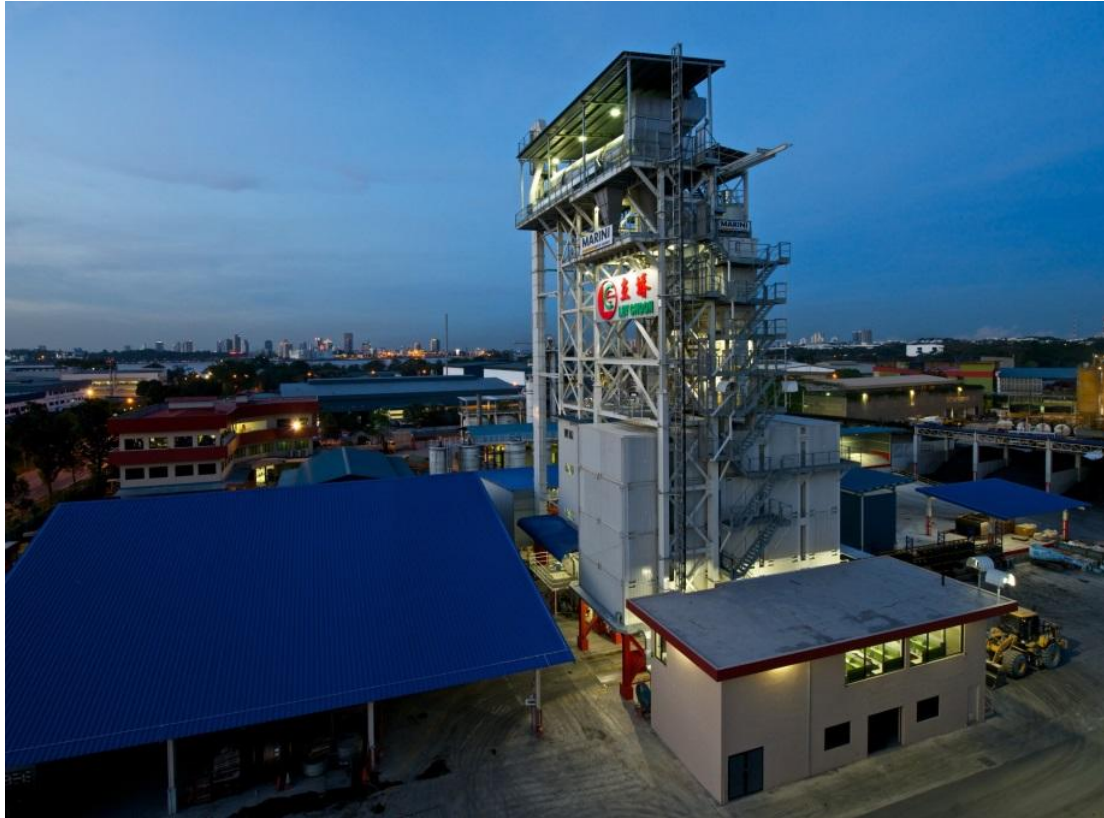
Ley Choon's 2nd asphalt recycling plant at No. 3 Sungei Kadut Drive
