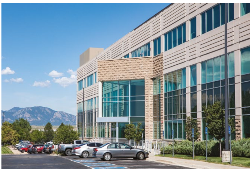
The improved operating performance mainly from The Plaza Buildings, The Westpark Portfolio and Westmoor Center (pictured), contributed to higher gross revenue for KORE in FY2022.
