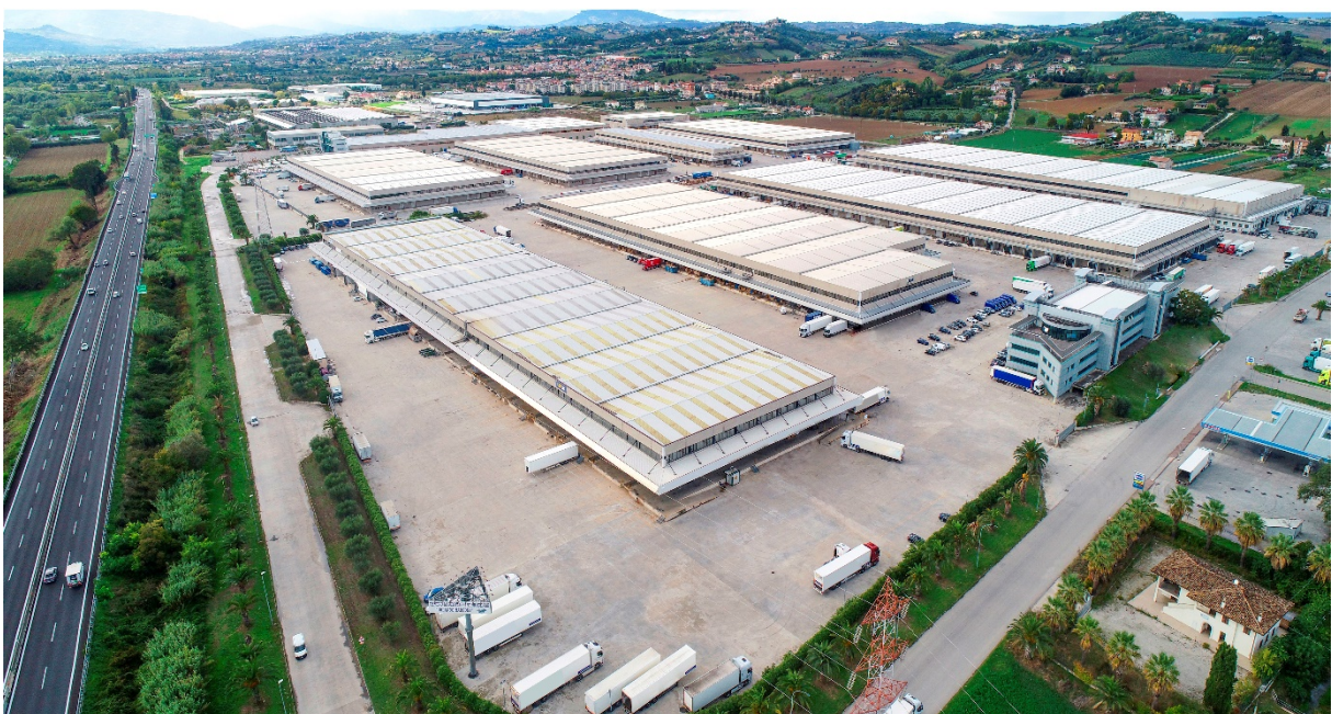
Centro Logistico Orlando Marconi, Montepandone, Italy
