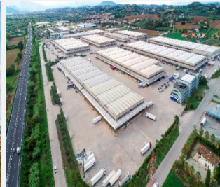
Centro Logistico Orlando Marconi Montepandone, Italy
