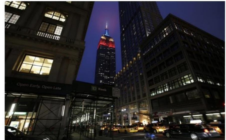
Heating buildings accounts for some 40 percent of New York City's carbon emissions. Mike Segar/Reuters
