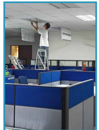
Replacing fluorescent lightings with energy-efficient LED lightings
