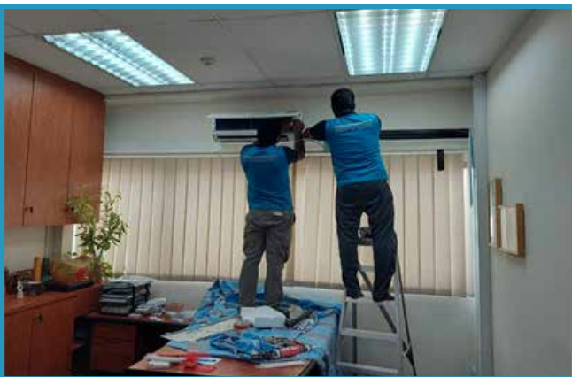
Replacing the air-conditioning units with Energy Efficiency 5x Green Ticks Mark
