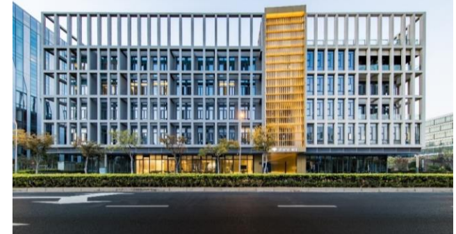
Shanghai Hongqiao Sincere Centre (Phase 2)
