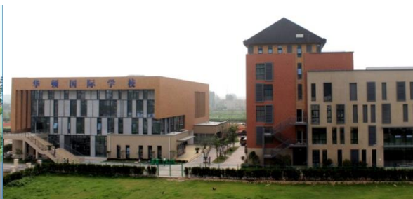
Wuxi Chiway School
