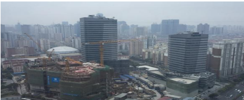
Overall Construction On Track
