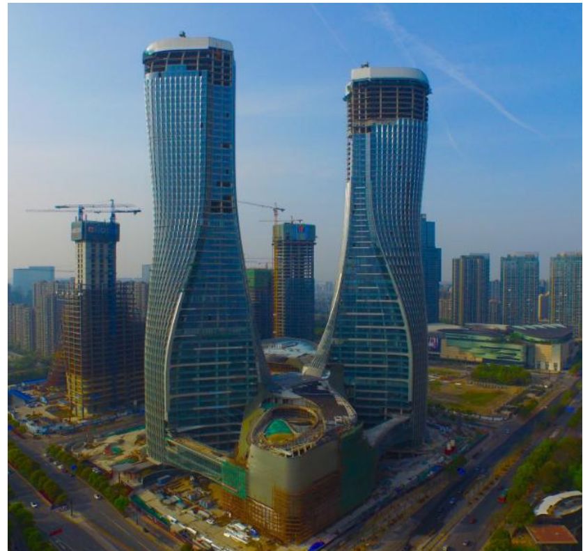
Curtain Wall Installation In Progress
