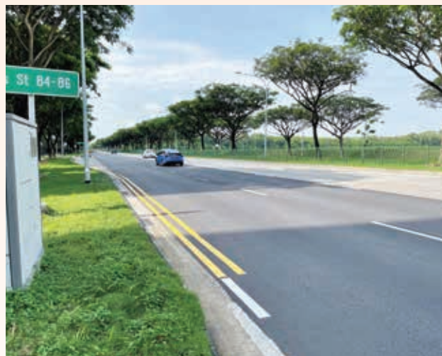
OKP is undertaking a road maintenance contract for North East sector.
