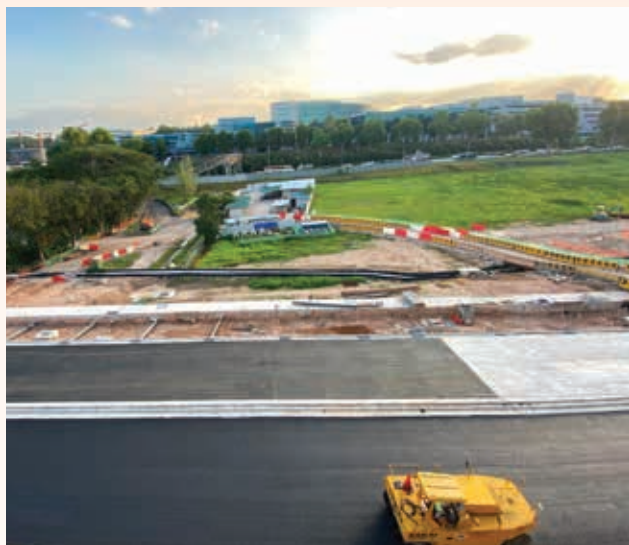
OKP has completed the construction of roads, drains and sewers at One-North Crescent and Media Link, and road demolition and reinstatement works at Portsdown Road.
