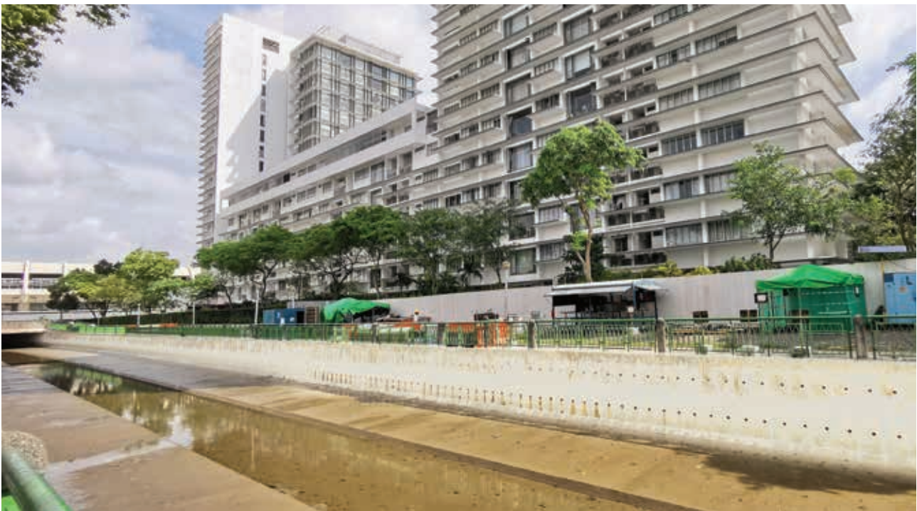
Improvement to roadside drains V Contract E5 (Yishun Avenue 1/6, Jalan Kembangan, Pasir Ris Estate and Hai Sing Estate areas) is an ongoing maintenance project.
