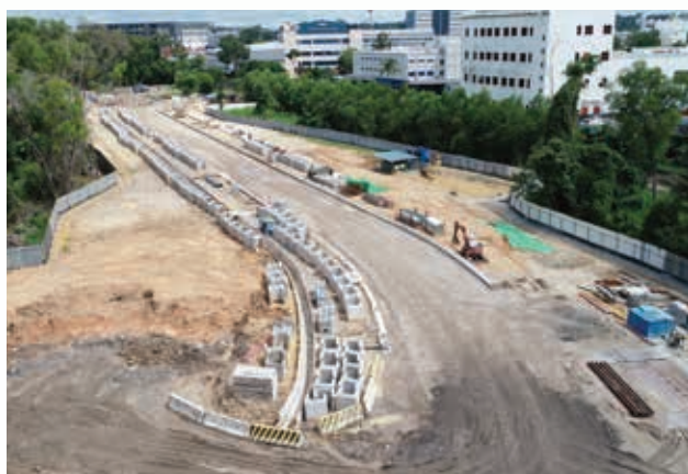
One of OKP's ongoing construction projects involves commuter and road infrastructure works in Pasir Ris and Loyang.
