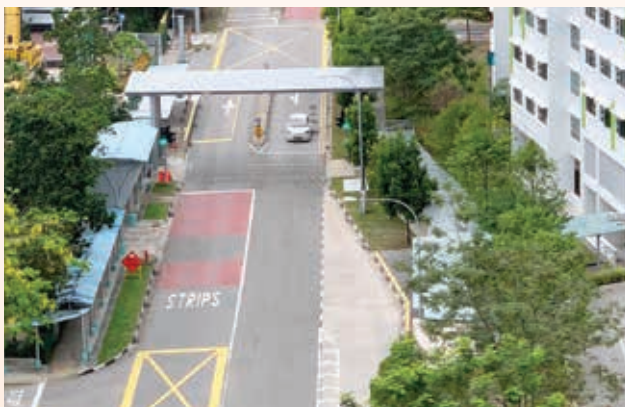
OKP is involved in constructing of covered linkways to Thomson-East Coast Line (TEL) Stage 1, 2 and 3 Stations (Woodlands Drive 14).
