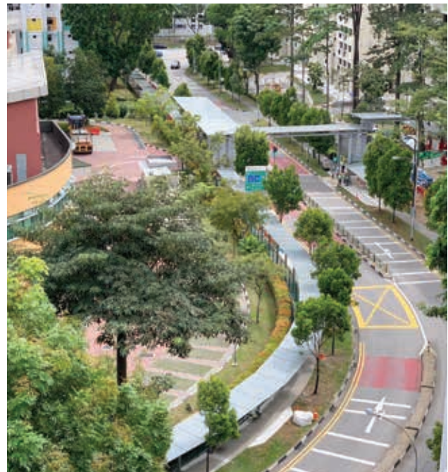
OKP is involved in constructing of covered linkways to Thomson-East Coast Line (TEL) Stage 1, 2 and 3 Stations (Woodlands Drive).
