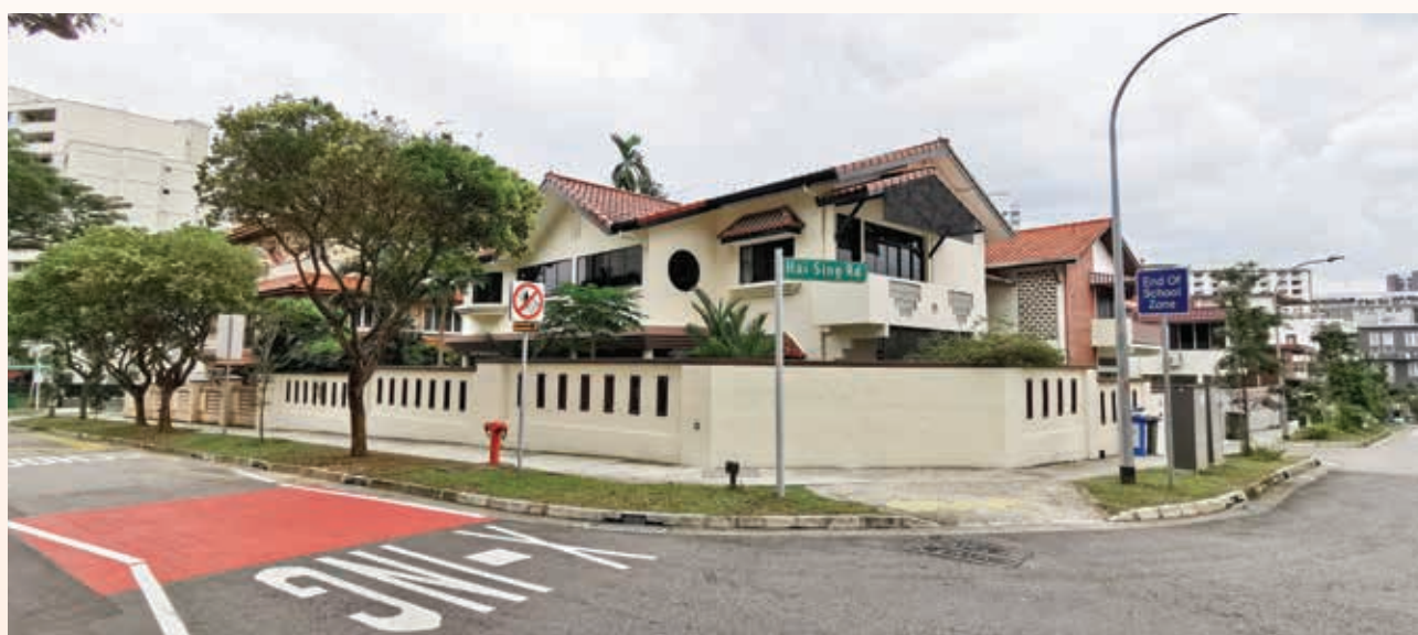
Improvement to roadside drains V Contract E5 (Yishun Avenue 1/6, Jalan Kembangan, Pasir Ris Estate and Hai Seng Estate areas) is one of OKP's ongoing maintenance projects.
