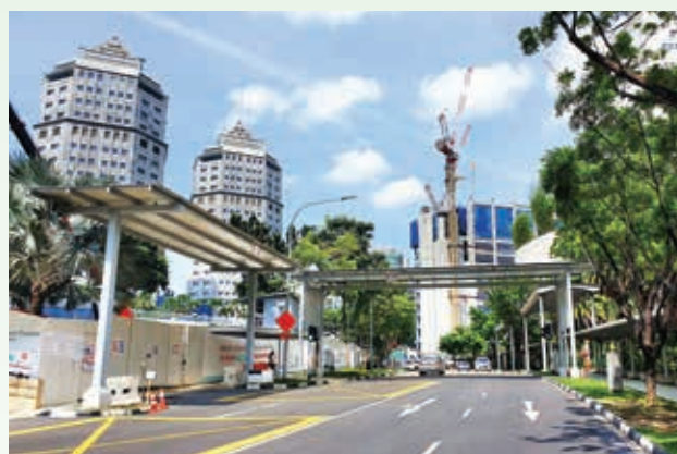
OKP is involved in constructing linkways under the Walk2Ride programme.
