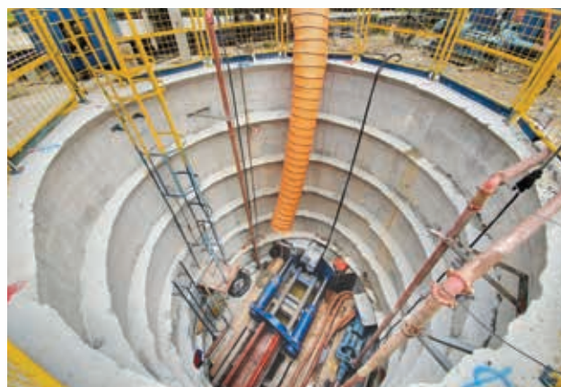
Overall view of jacking shaft in the proposed construction of new infrastructure at Tukang Estate.
