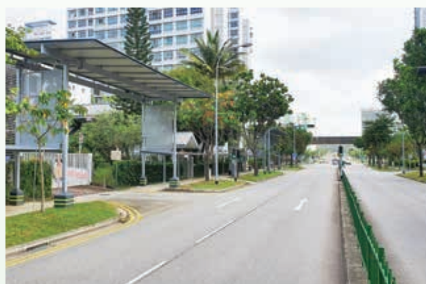
Under the Walk2Ride programme, OKP has completed the covered linkway at Damai.
