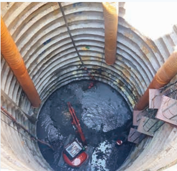
The construction of link sewers from the Deep Tunnel Sewerage System phase 2 project – schedule III contract 1 (Jalan Buroh/Tanjong Kling Road) is currently being undertaken by OKP.
