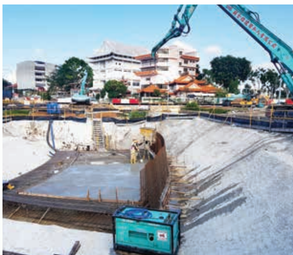
OKP is undertaking the project for the widening of Tampines Road between Kallang Paya Lebar Expressway (KPE) and Tampines Avenue 10.
