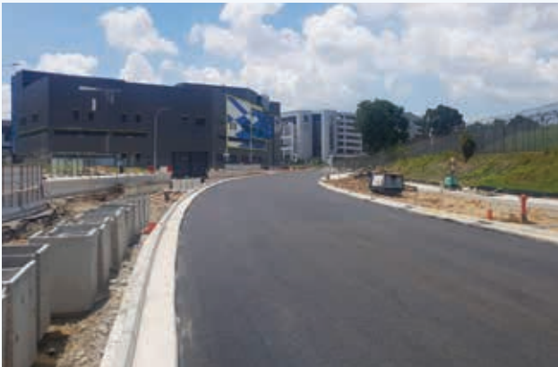
The widening of Tampines Road between Kallang Paya Lebar Expressway (KPE) and Tampines Avenue 10 is an ongoing construction project.
