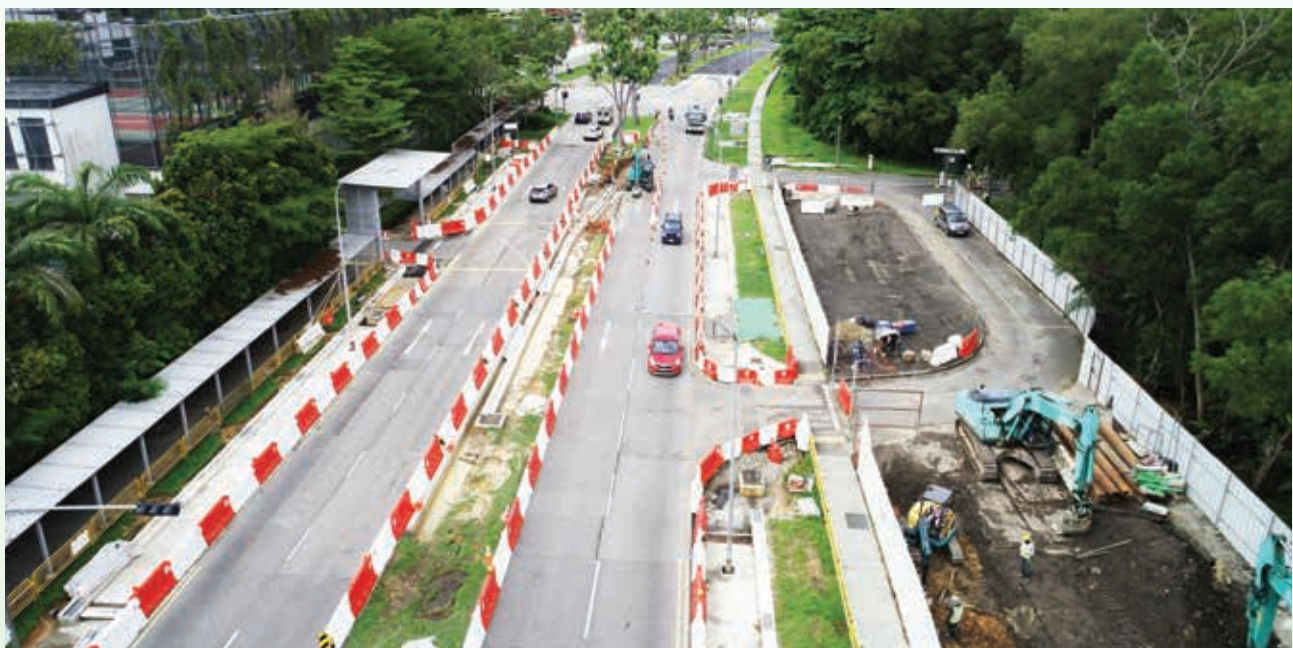
OKP is carrying out commuter and road infrastructure works in Pasir Ris and Loyang.
