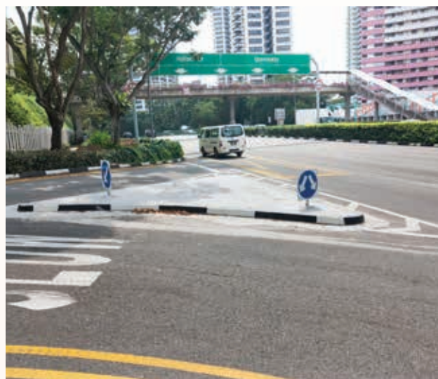
OKP is undertaking a term contract for road related facilities, road structures and road safety schemes for East Sector, one of which is at Farrer Road.
