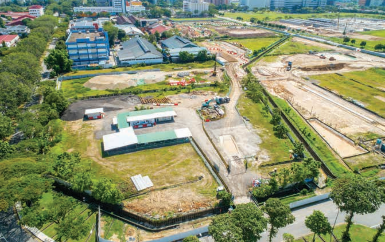
An overview of the site for the proposed construction of new infrastructure at Tukang Estate, which is one of OKP's projects.
