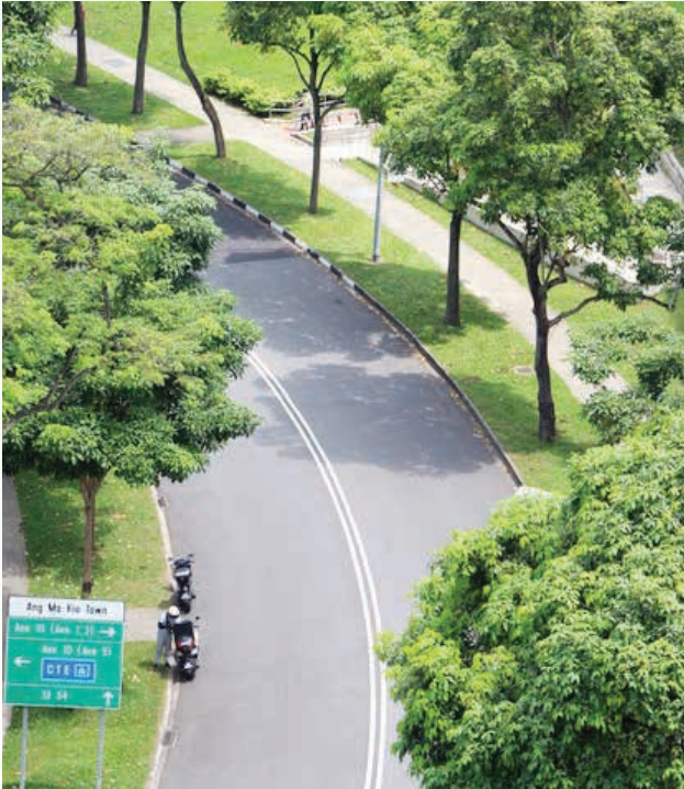
OKP is involved in a road maintenance contract for North East Sector at Ang Mo Kio.
