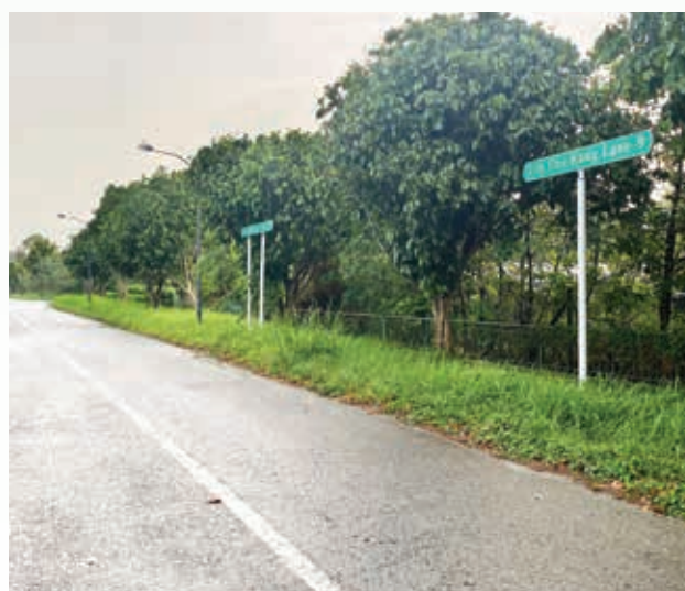
OKP completed the proposed sewers in Lim Chu Kang area - contract 2.
