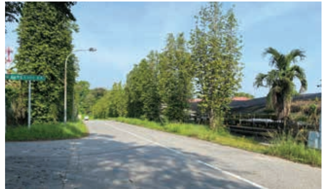
OKP is involved in the proposed sewers in Lim Chu Kang area - contract 2.
