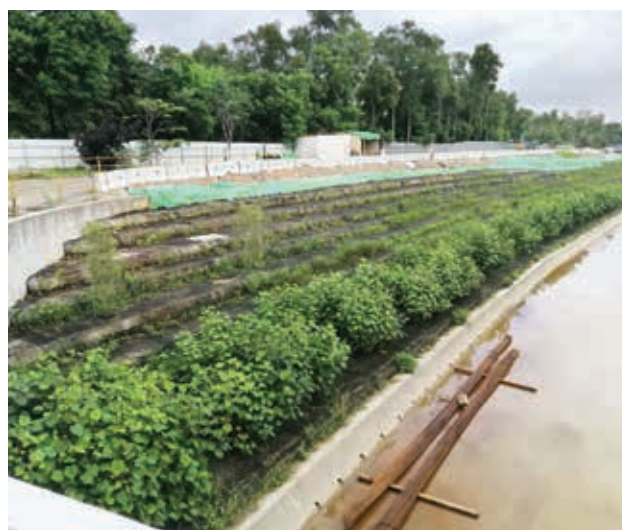
One of OKP's construction projects involves improvement works for Sungei Tampines (Tampines Avenue 7 to Tampines Expressway).
