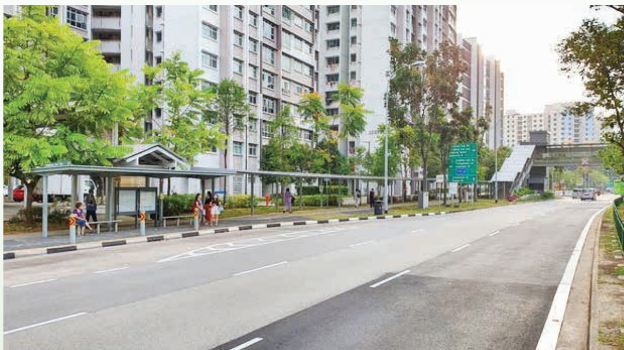
The covered linkway at Cheng Lim Road is one of OKP's projects under the Walk2Ride programme.
