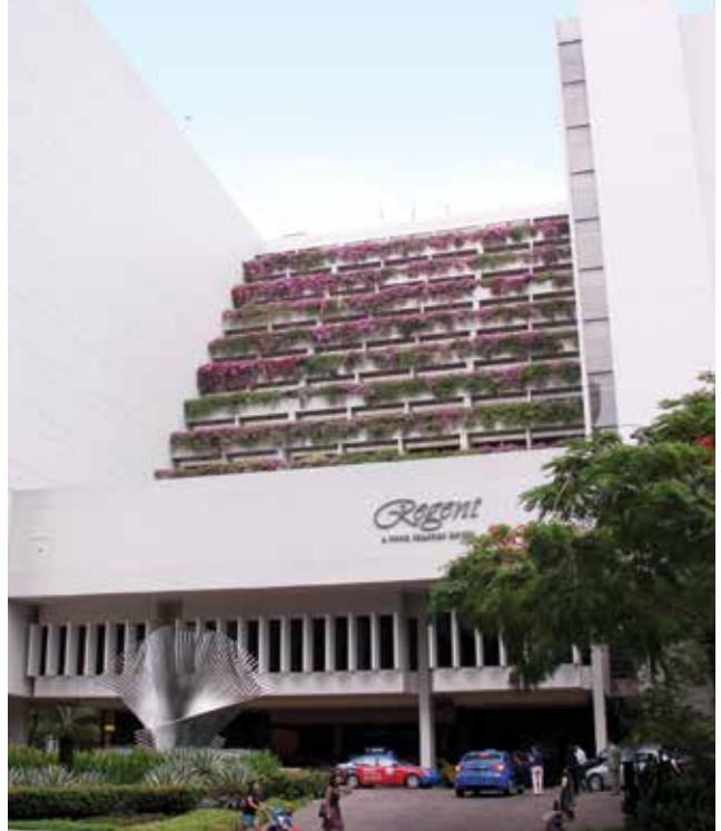
R&R project at Regent Singapore
