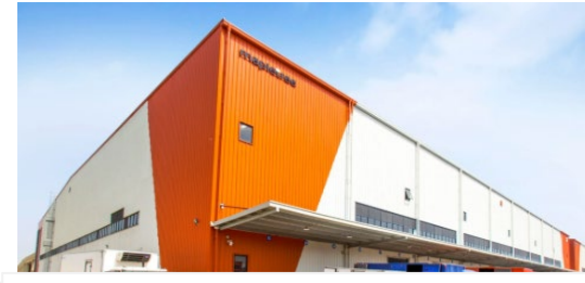
Mapletree Wuxi New District Logistics Park, China
