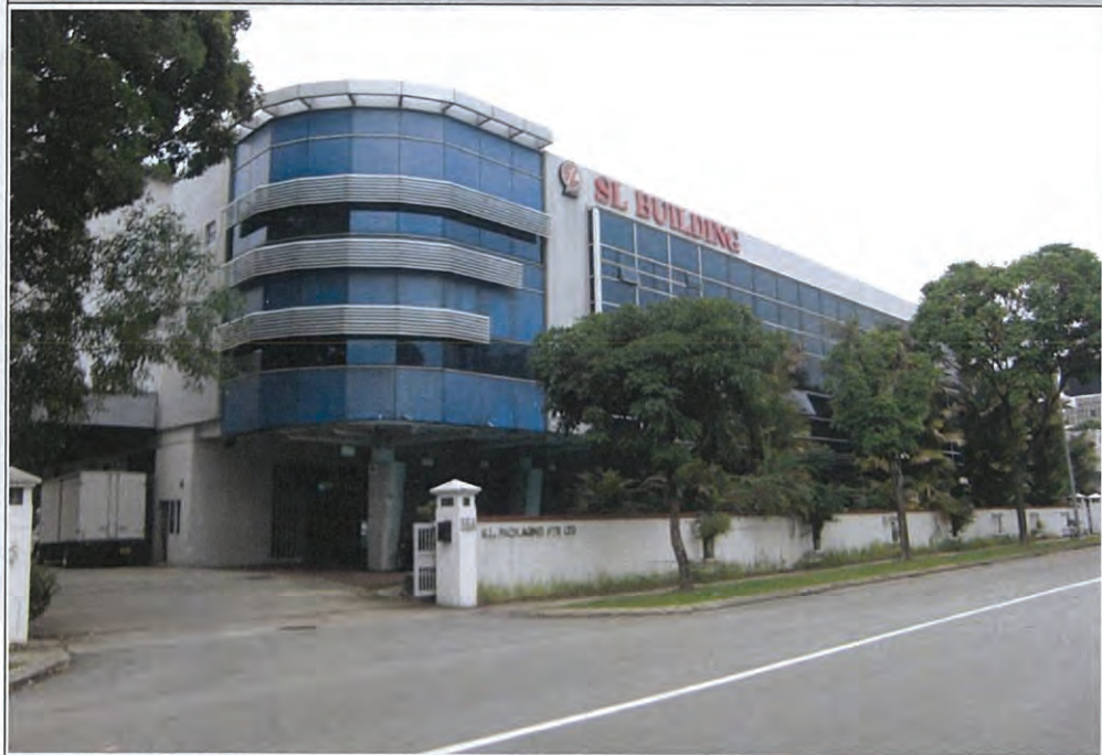
Figure 5.0 View of the Property
