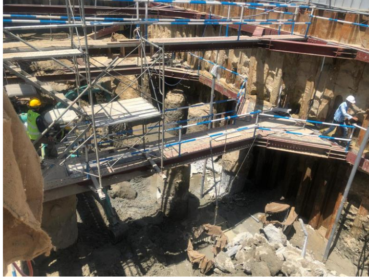
Soil Excavation and piling works in progress.
