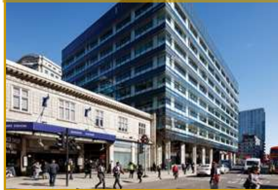
Asset Refurbishment @ Aldgate House
