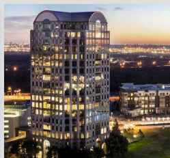
TOWER 909 Dallas, Texas
