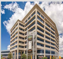
VILLAGE CENTER STATION I Denver, Colorado
