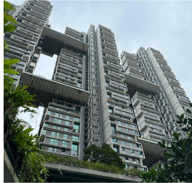
R&R to 6 HDB blocks at Dawson Road
