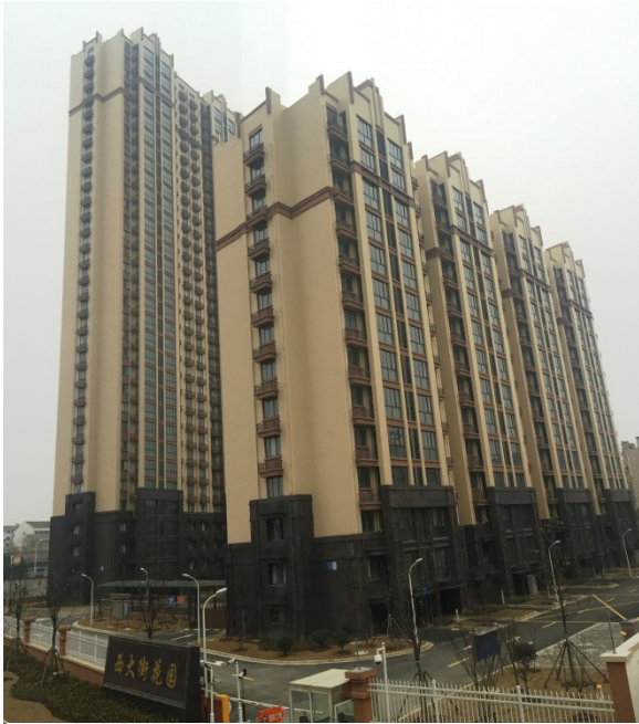
Residential Build-and-Transfer Project, Jiangyin
