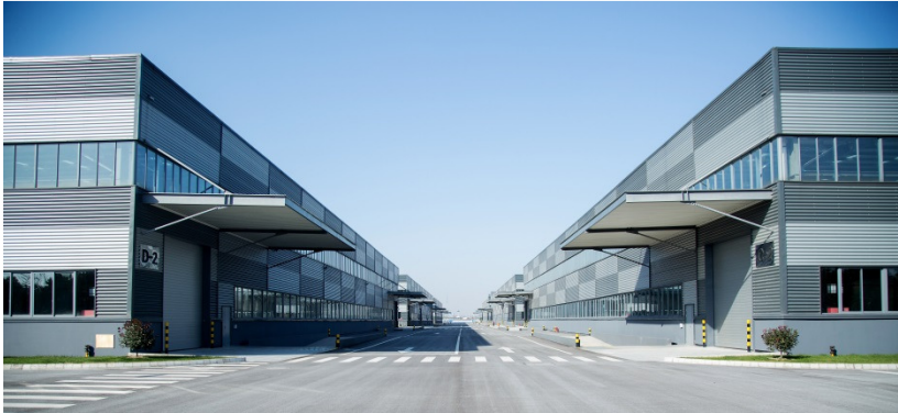
Changshu Fervent Industrial Park, Jiangsu
