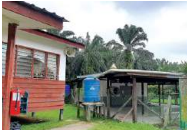
Rainwater harvesting tank for office and housing
