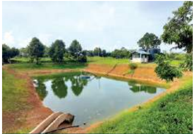
Rainwater harvesting pond installed for the nursery
