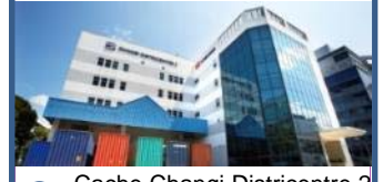
8 Cache Changi Districentre 2 3 Changi South Street 3
