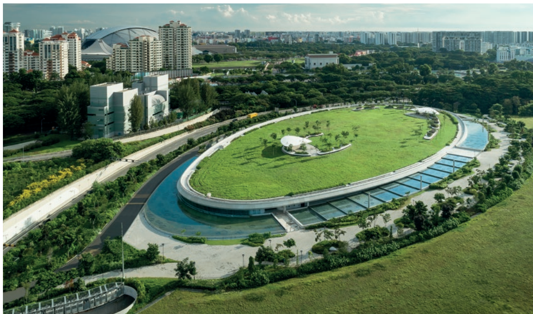
Keppel Marina East Desalination Plant, Singapore's first large-scale, dual-mode desalination plant which is capable of producing 137,000 m 3 of fresh drinking water per day, contributes to Singapore's water security amidst increasing rainfall uncertainty caused by climate change.
