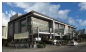
Siloam Hospitals Bali
