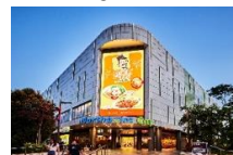
Northpoint City North Wing 2017
