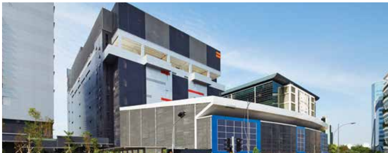
Hi-Tech Building, 26A Ayer Rajah Crescent
