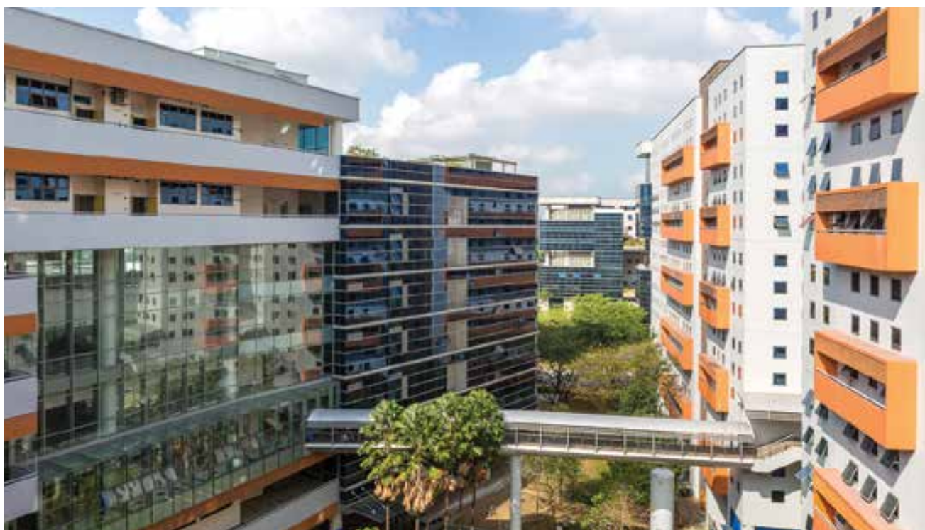
Stack-up/Ramp-up Buildings, Woodlands Spectrum
