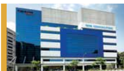
29 TATA COMMUNICATIONS EXCHANGE
