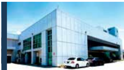
38 19 CHANGI SOUTH STREET 1
