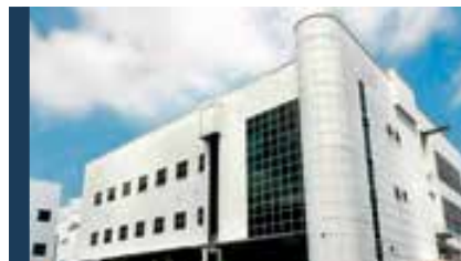
39 65 TECH PARK CRESCENT
