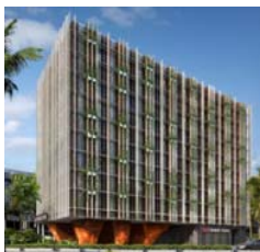
Crowne Plaza Changi Airport Extension (100% stake) 1
