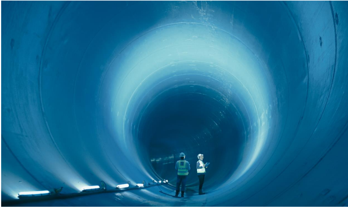
Tuas Corrosion Protection Lining
