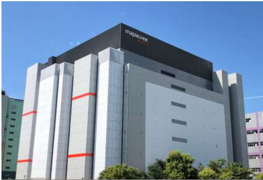
7 Tai Seng Drive (after upgrading into a data centre)
