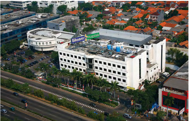
Siloam Hospitals Kebon Jeruk
