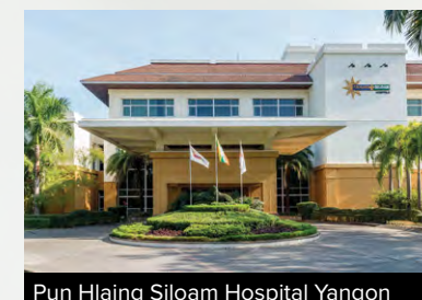
Pun Hlaing Siloam Hospital Yangon
