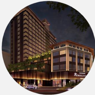
4 Night Lighting @ Podium
