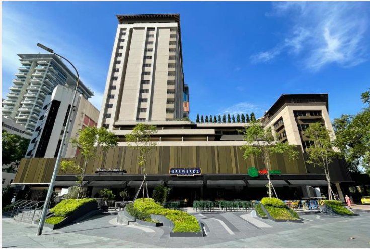
New Ribbon Cladding
