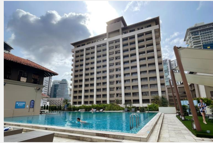
Removal of Existing Planter Boxes
