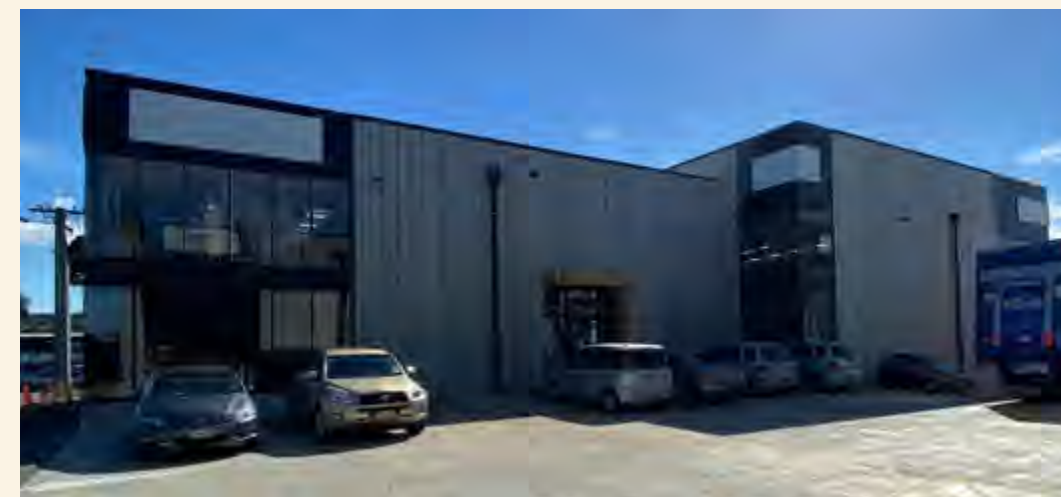
NEW ZEALAND WAREHOUSE
