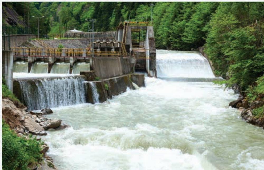
HYDROELECTRIC POWER PLANT
