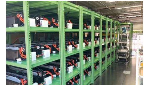
Large-capacity sweep energy storage system that uses electric car batteries
