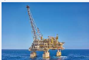
Wheatstone LNG Project, Australia Source: Chevron Australia
