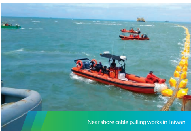
Pipe conduit pullback operation in Yulin, Taiwan
